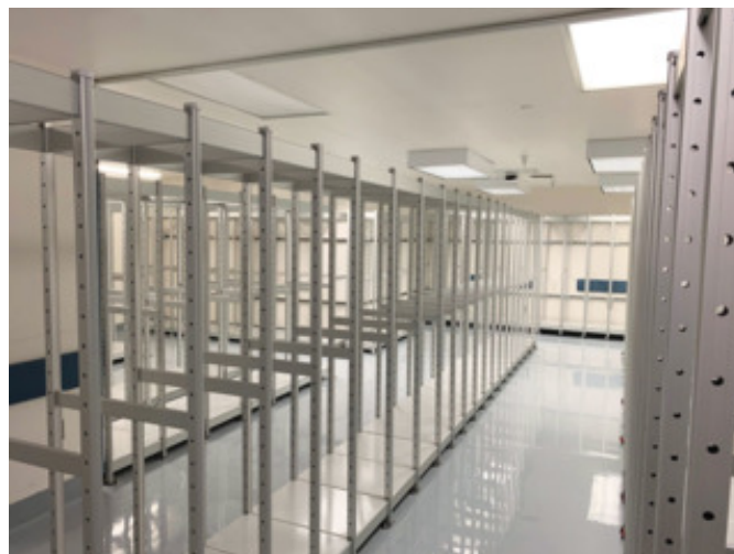
UCSF: Construction under way!
