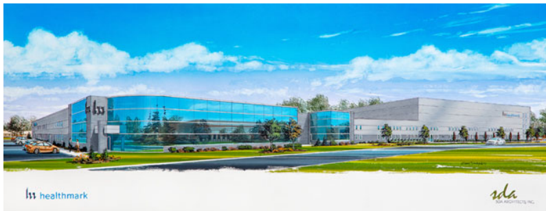
New construction of the Healthmark Industries Headquarters.
